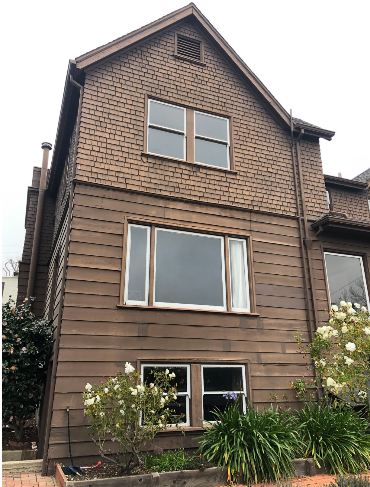
Fig.22 – 2119 Marin Ave. – West side, rear
