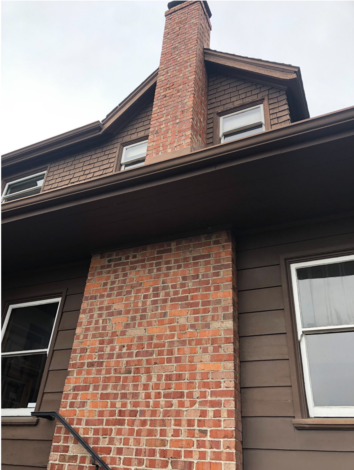
Fig.21 – 2119 Marin Ave. – Chimney at west side
