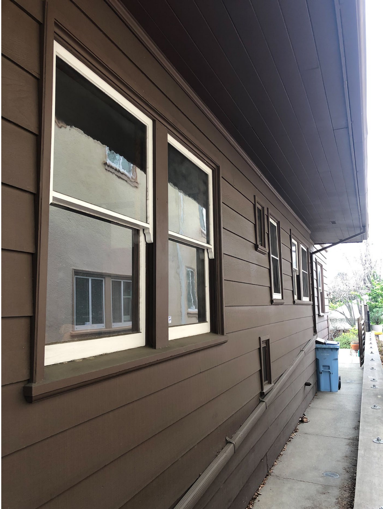
Fig.23 – 2119 Marin Ave. – East side
