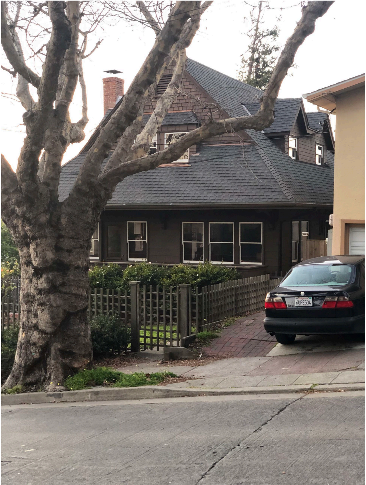
Fig.13 – 2119 Marin Ave. – Front and part east side
